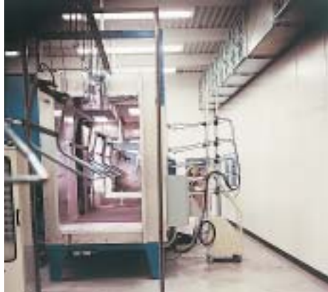
Powder coating application room.
