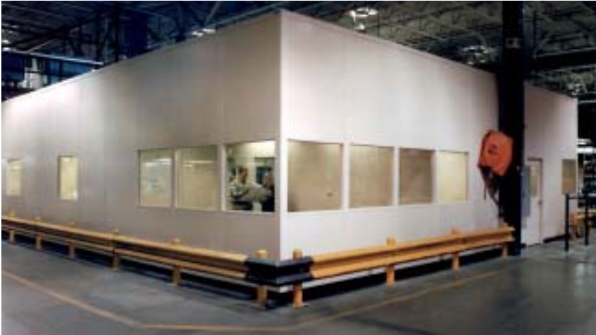
Office complex with protective guard rail.
