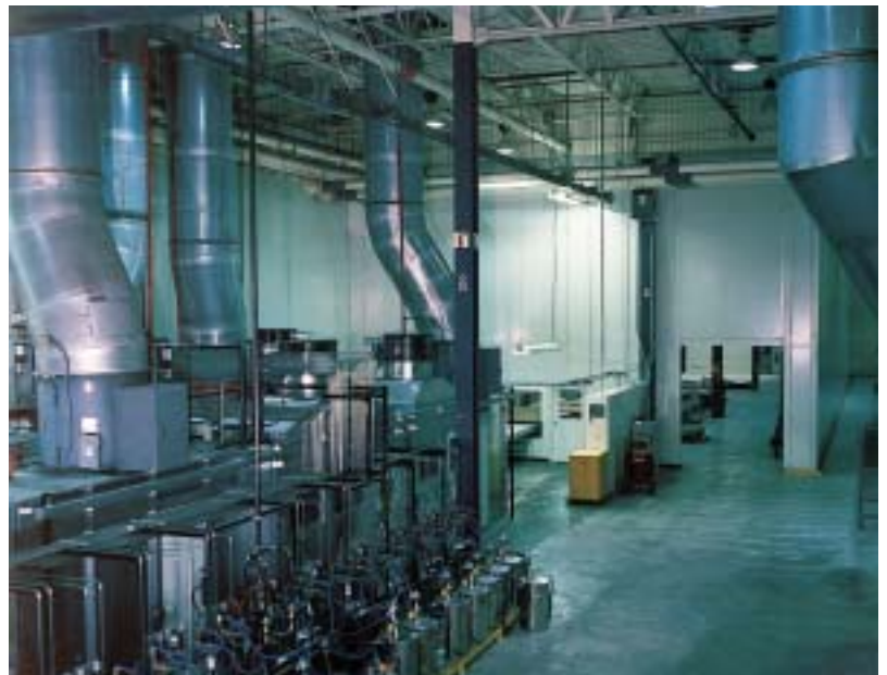
Finishing system enclosure enables control of temperature, humidity and particulates.
