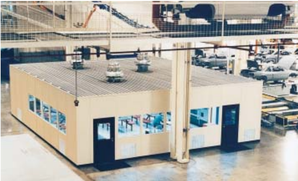
Breakroom in an automotive manufacturing plant.
